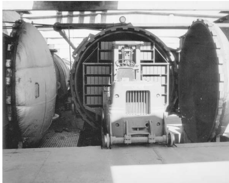
Figure 2-7 Loading racks of fresh units into an autoclave for high-pressure steam curing. (Photo courtesy PCA.)
